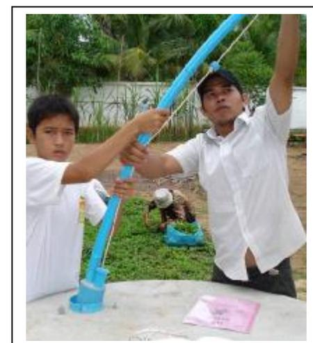
Figure 11 Installing the guide box and riser pipe
